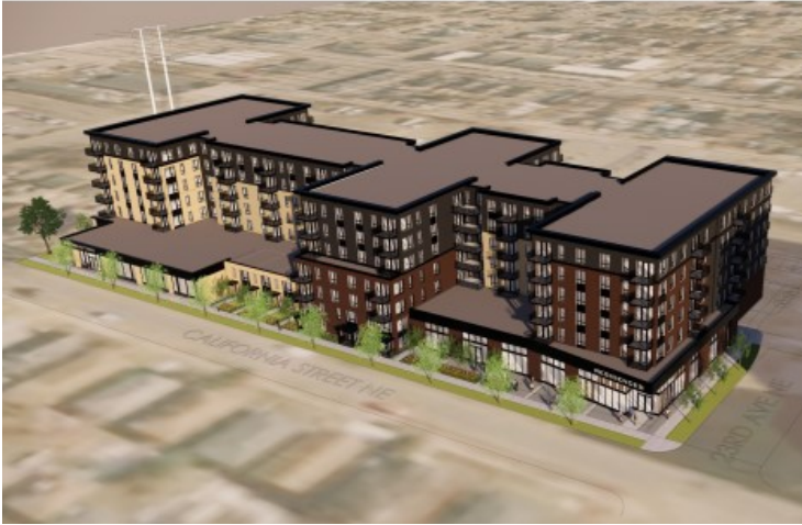
Rendering of development proposal for 2301 California Street NE from LS Black Developers
